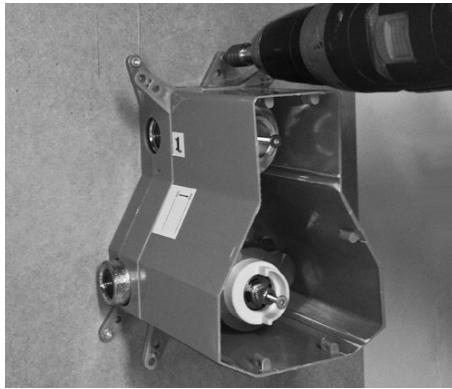
4. Affix the mixer to the structural rear wall using four screws.
