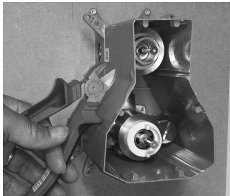
9. Once the wall has been finished off the casing can be trimmed to size.
