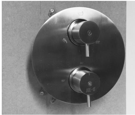
12. Affix the thermostat knob and tighten the socket-head screw with a hex key, making sure that the indicator is pointing downwards. Your JEE-O slimline mixer TH is now ready for use.
