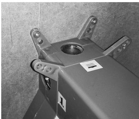
5. There are three outlets at the top of the mixer. The stopper included in the bag of screws can be used to cover any of these outlets, if desired.
