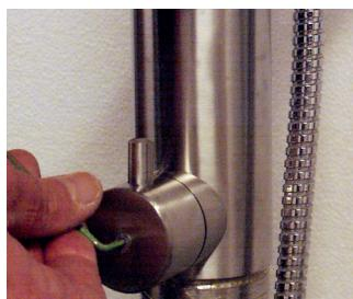
**4. Detach the thermostat knob by removing the socket-head screw.**
