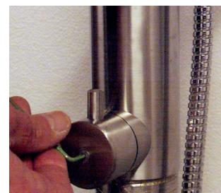
**6. Reassemble the thermostat knob and tighten the socket-head screw with a hex key, making sure that the indicator points upwards (O2TH) or downwards (slimline).**
